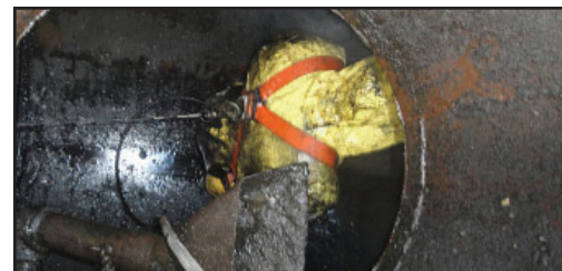
ABOVE GROUND STORAGE CLEANING
